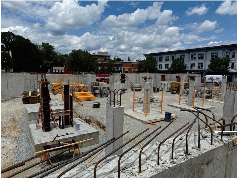
July 8: footings and foundations.
