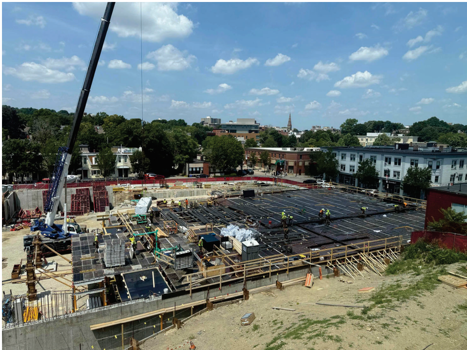
July 24: view of site.
