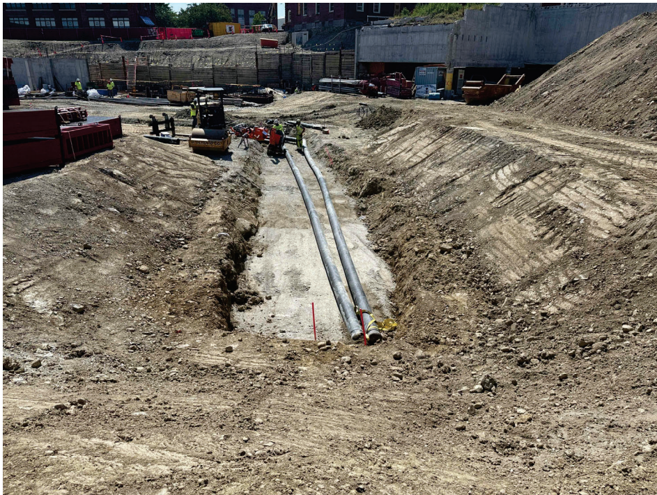
July 8: geothermal lines.
