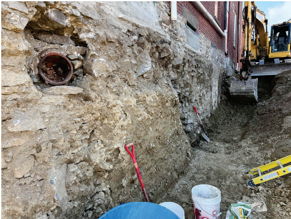
July 17: Historic Building foundation exposure.
