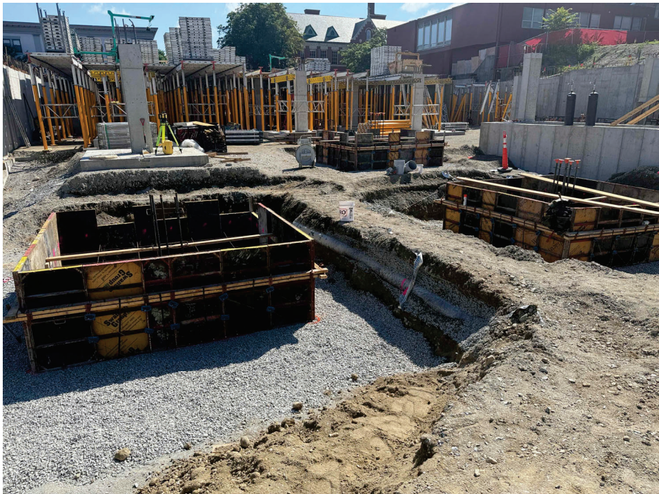
July 15: footings and foundations.
