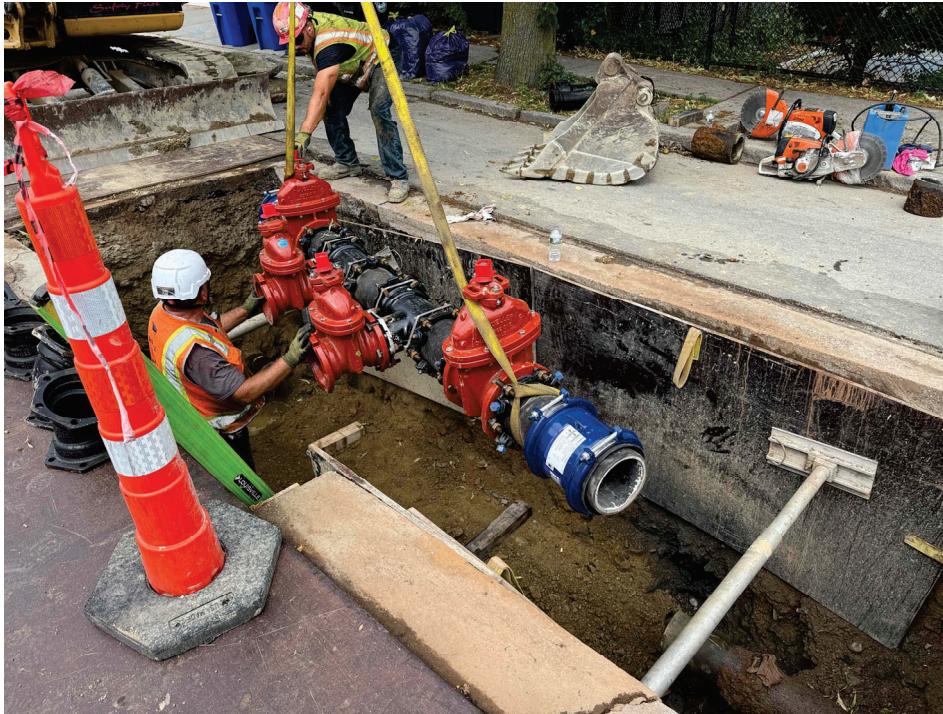
July 2: street utility work.
